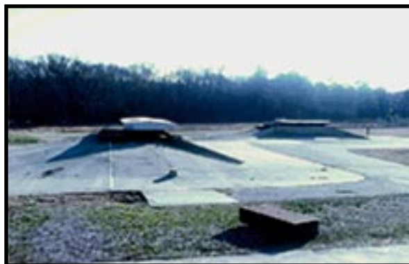
View of burning pans on a secondary containment pad. Note that the pads do not appear to have berms around them.
