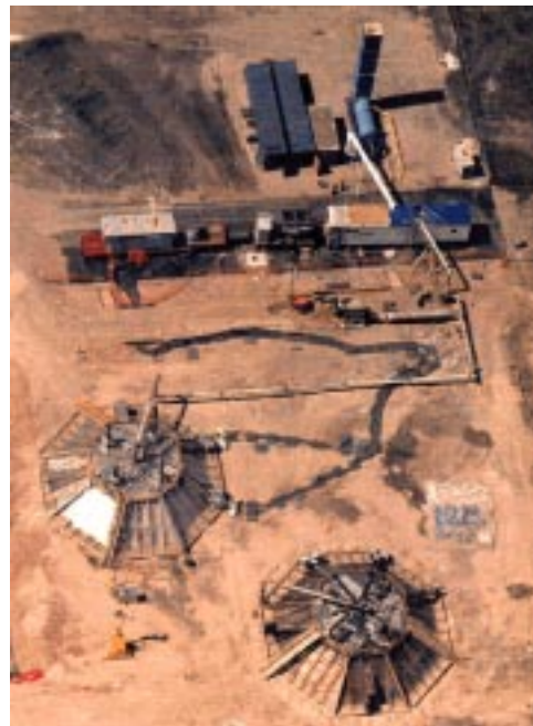
In-situ vitrification hoods.
